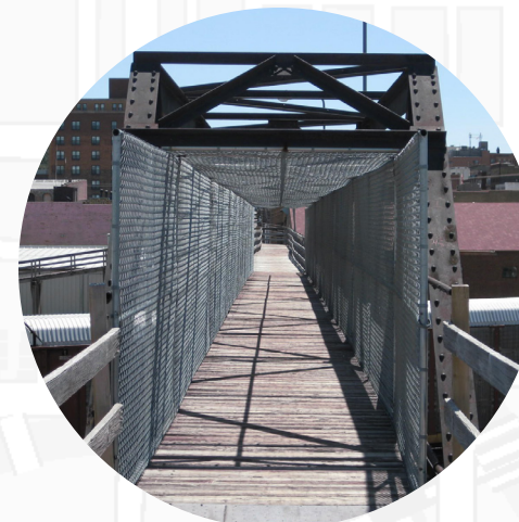
Pedestrian bridge over rails near site
