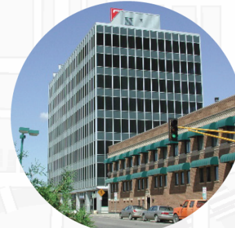
View of the existing building on site
