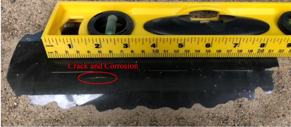
Figure 69. Visual inspection result for the steel pipe sample at 60th day.
