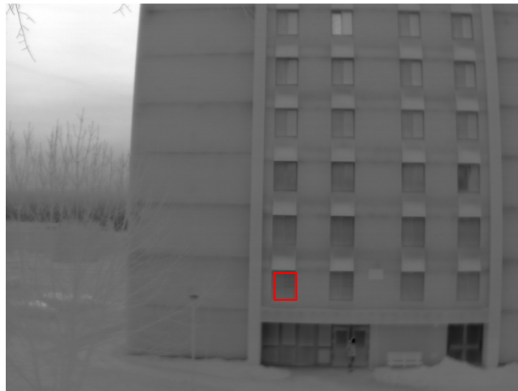
Figure 4.6. Thermal image of East side of the Thompson Hall – December 21.
