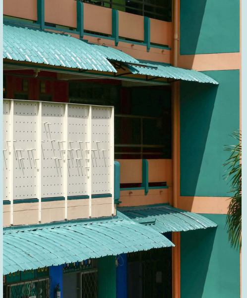
Image of school building Figure 2.01
