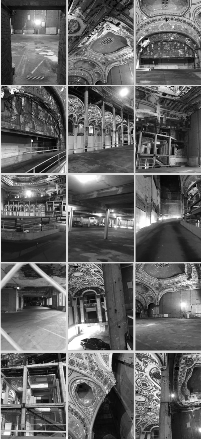
Michigan Theater - Interior Condition
