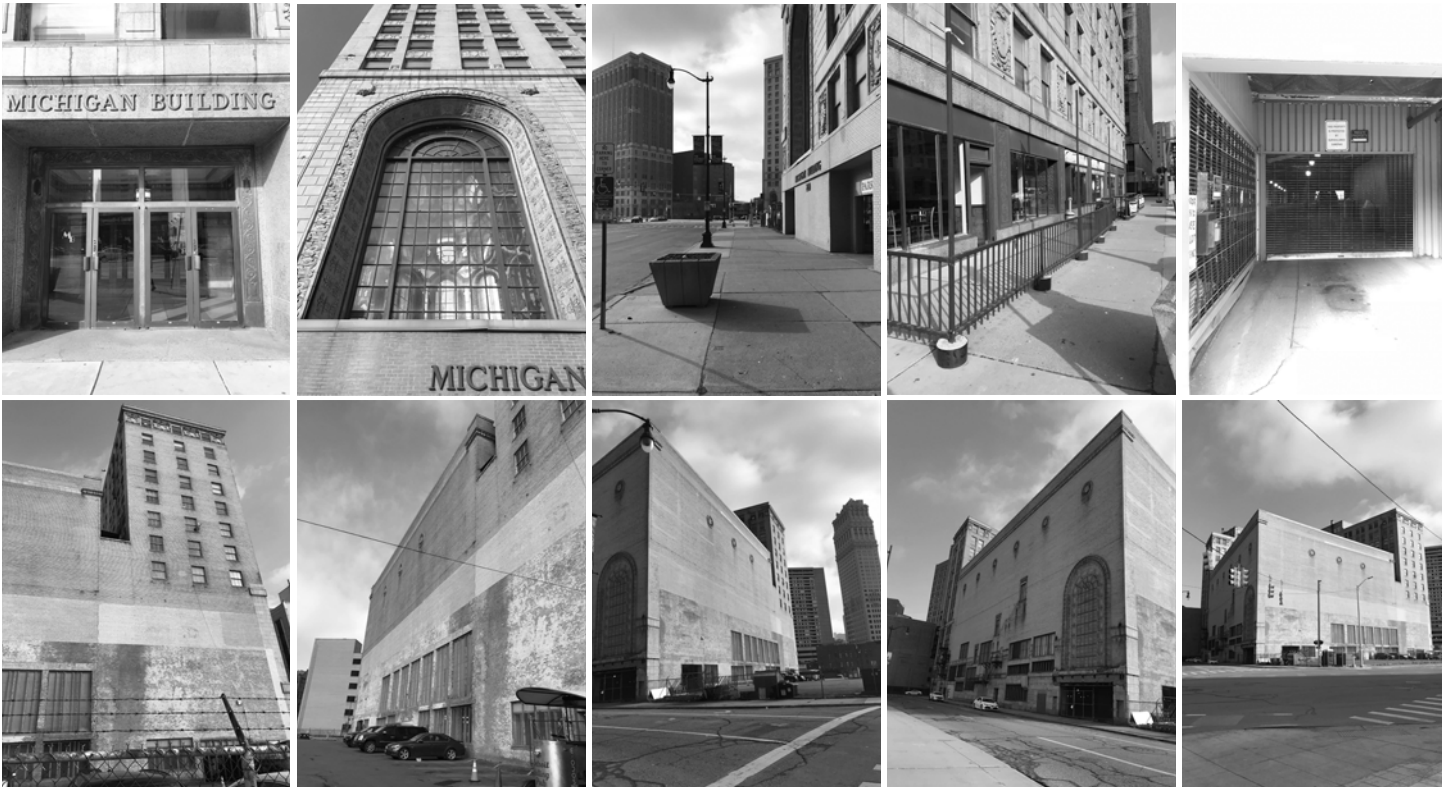
Fig. 122: Michigan Theatre - Exterior Condition
