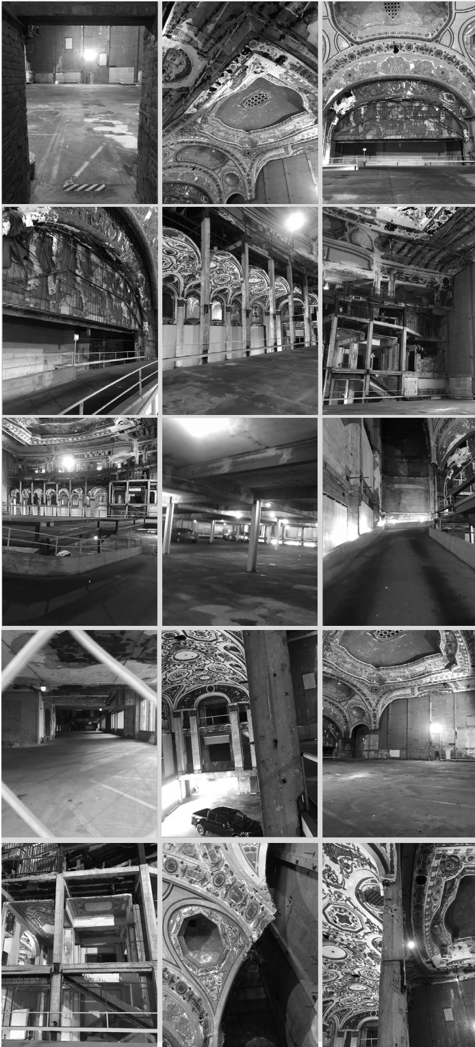
Fig. 121: Michigan Theatre - Interior Condition
