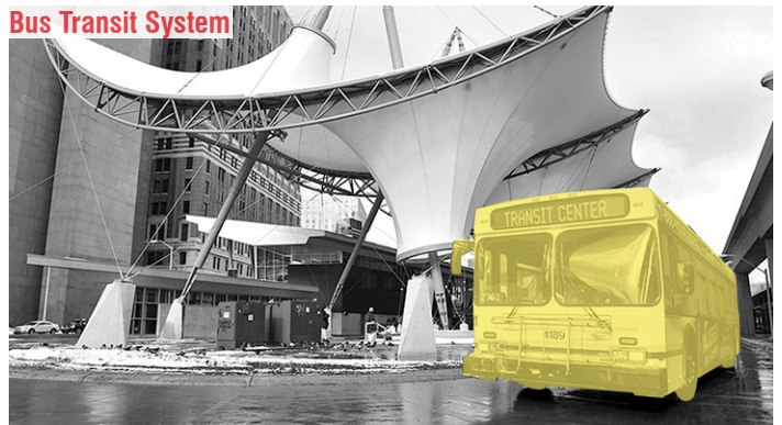
Fig. 136: Detroit Bus System: Rosa Parks Transit Center
