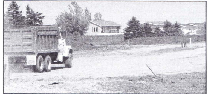
Work began on the new Wild Rice addition development in spring 2007.
