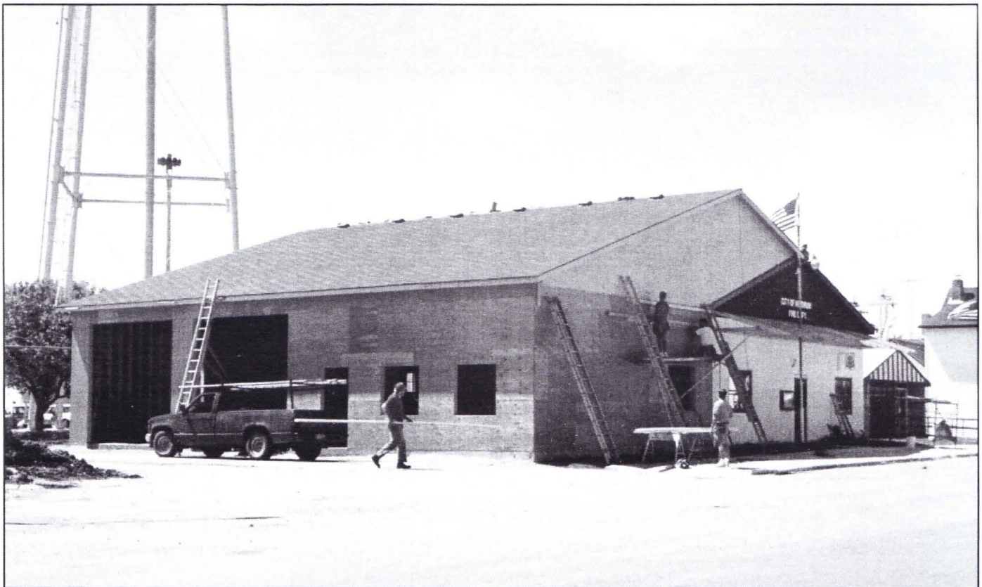
Doubling the size of the Hendrum Fire Hall in 1997.
