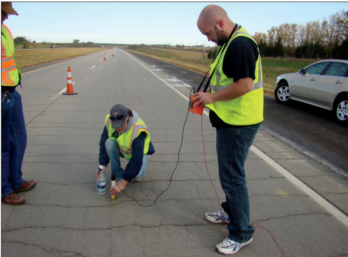
Half-cell potential measurements of CRC pavement in South Dakota
