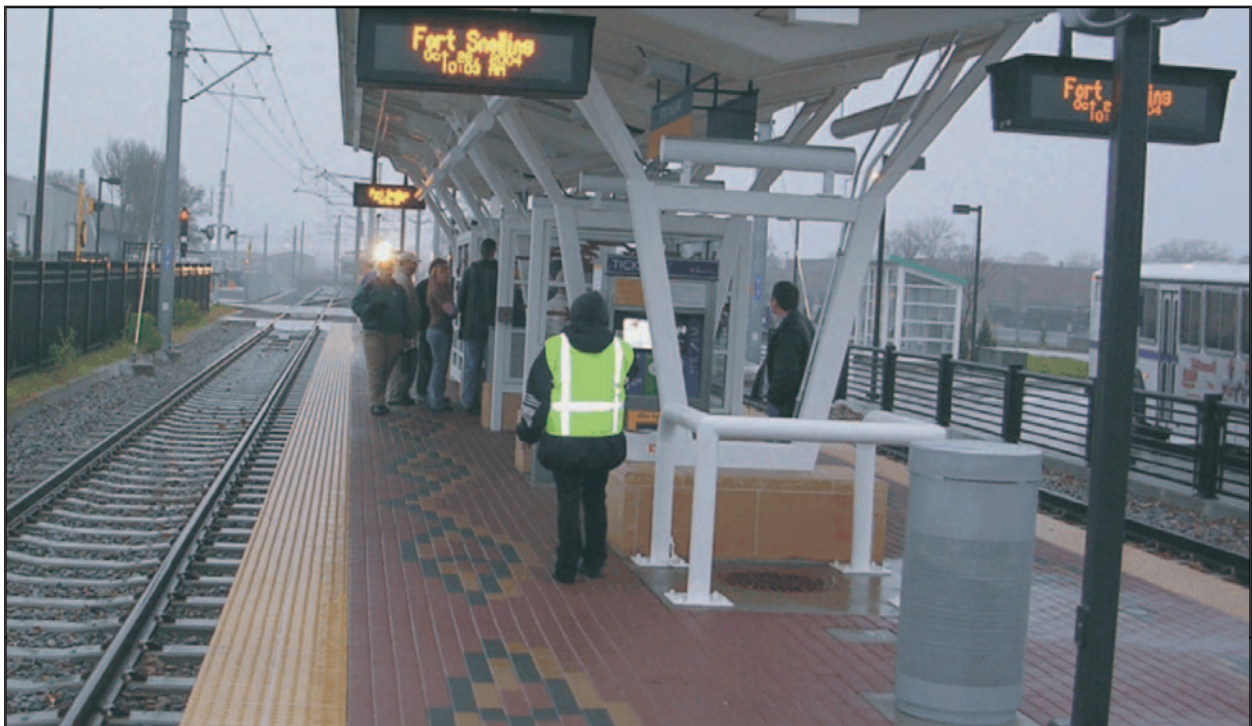
Students rode Metro Transit's Hiawatha Line, a new light rail transit system. (Minneapolis, MN)
