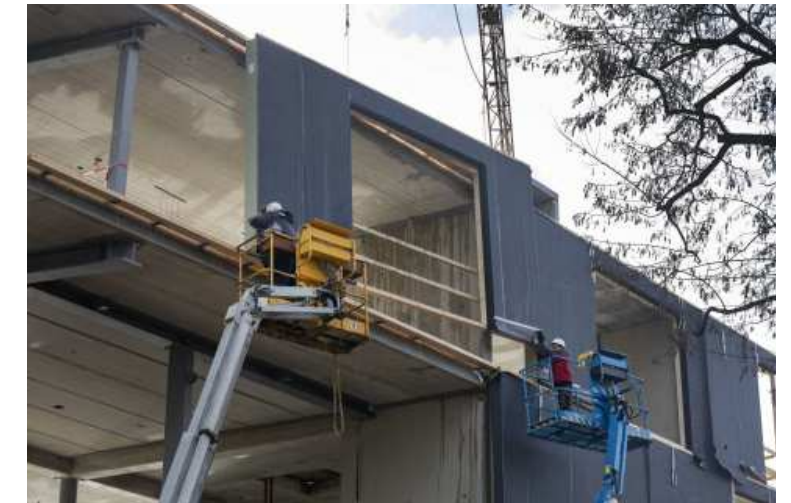
Figure 27 : SIP Installation | APA foto
