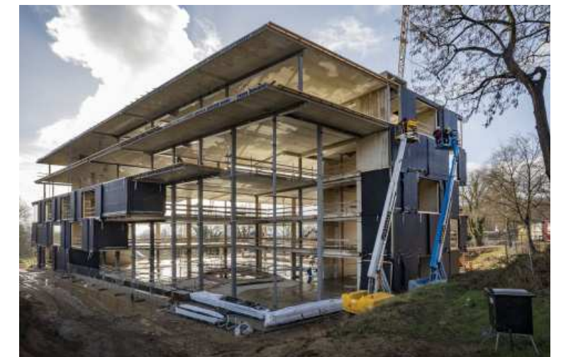
Figure 28 : Building Structure | APA foto
