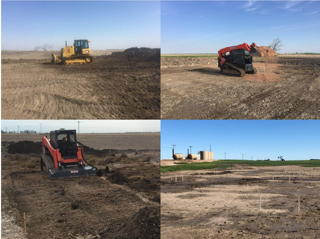
Figure 2.3. Top left image showing the removal of A-horizon using a bulldozer. Top right depiction of how amendments were applied to the treatment sub-plots (amendment pictured here is gypsum). Bottom left shows tilling in the amendments to the B-horizon. Bottom right shows a plot after the reclamation process with plots staked and ready for planting of cover crop.
