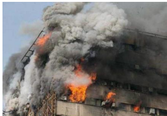
Plasco building, Tehran (2017) (Credit: Antonio Bilotta)
