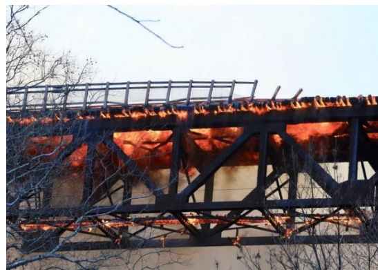
Railroad bridge fire, Pennsylvania (2018) (Source: Fox News)
