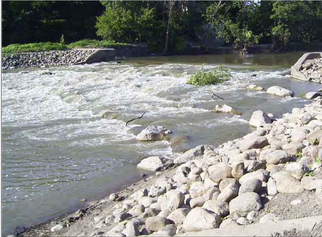
Picture 8 - Example of a rock-rapids fish passage structure at North Dam, Red River of the North, Fargo, ND. Project completed in 2002.
