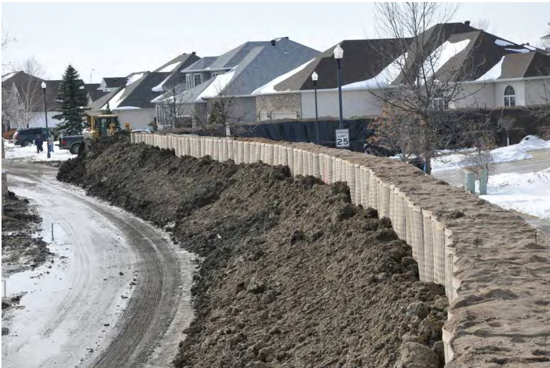
Picture 6 – Sand filled barriers were backed with clay and used as a second line of defense after the sandbags in 2009
