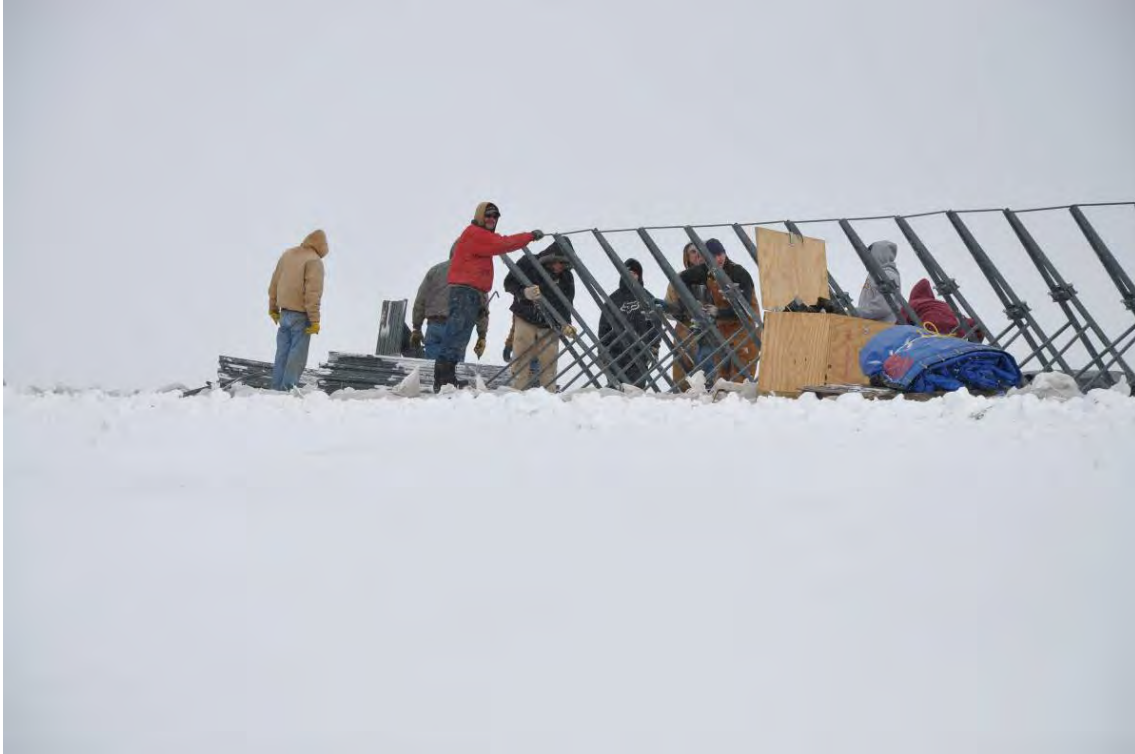
Picture 3 – Citizens set up steel frames to hold back the water in 2009
