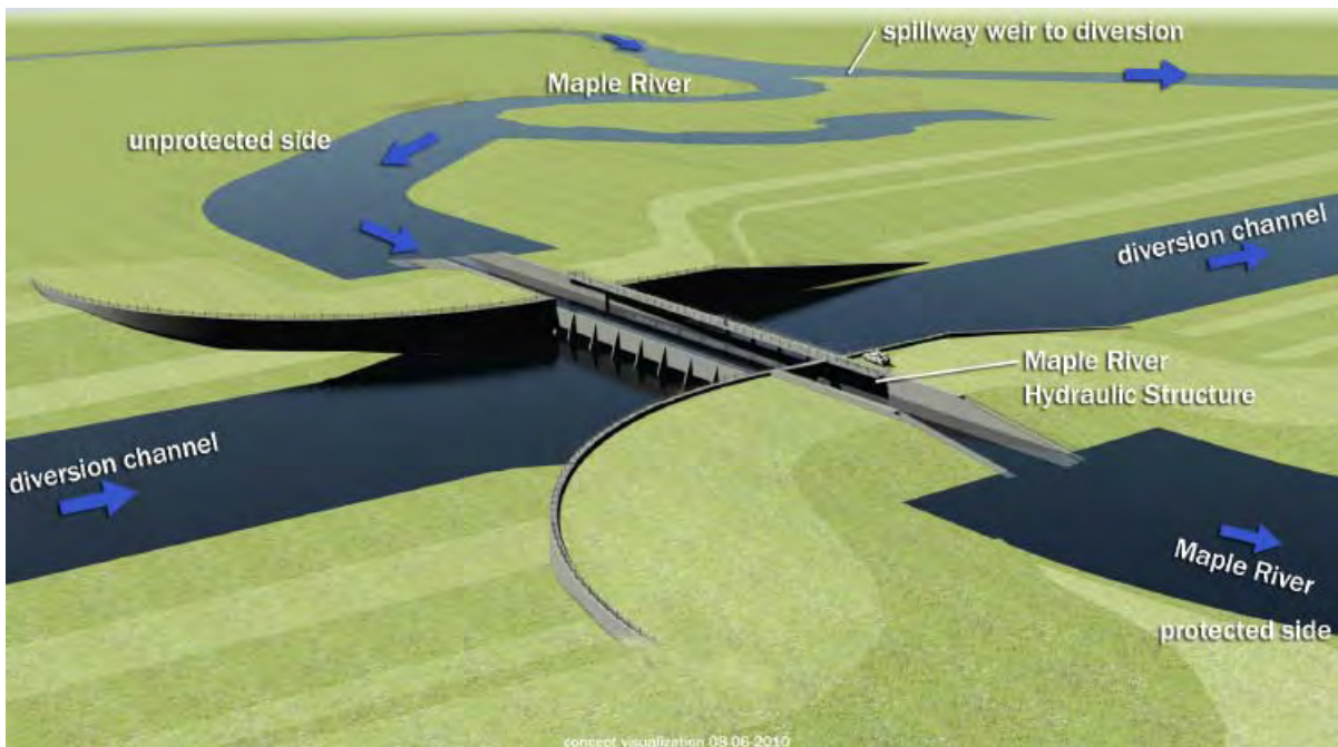
Figure 34 - Maple River Aqueduct visualization
