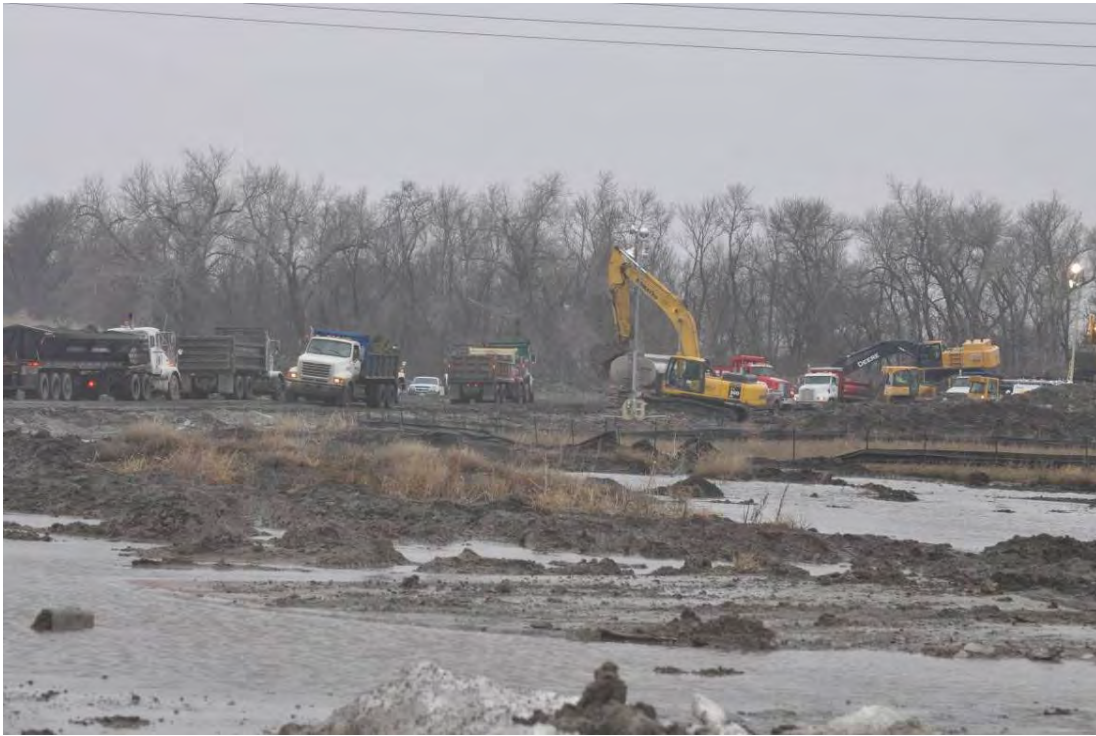
Picture 5 – Agricultural lands, sport facilities, and public areas were dug up for levee material in 2009
