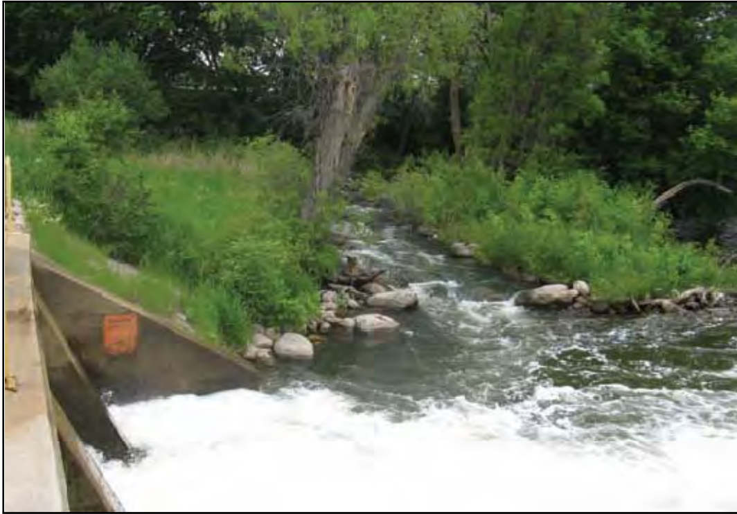
Picture 10 - Example of a fish bypass channel at a dam on the Otter Tail River near Fergus Falls, MN. Project completed in 2002. Photo and information source: Aadland 2010.
