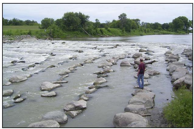
Figure 2. Example of a Red River fish passage project at Riverside Dam, Grand Forks, ND. Proposed project would generally look similar to this example.
