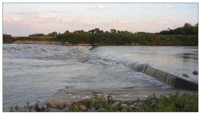
Figure 3. Drayton Dam on the Red River of the North, just north of Drayton, ND. Photo from September 18<sup>th</sup>, 2008 at a river discharge of approximately 6,400 cfs.
