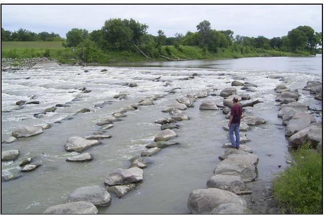
Figure 4. Example of a rock rapids fish passage project at Riverside Dam, Grand Forks, ND on the Red River of the North.
