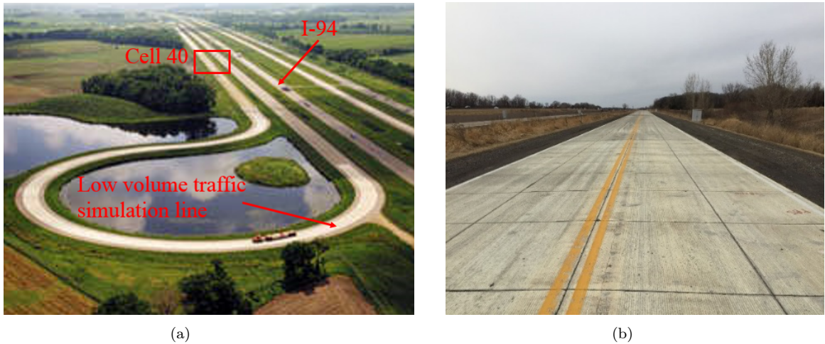
Figure 1: MnROAD Facility at MnDOT. (a) the road sections managed by the MnROAD Facility; (b) the concrete road section.
