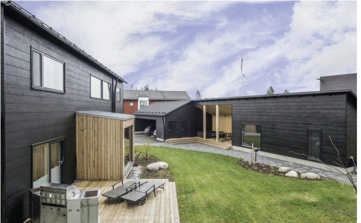
FIGURE 20 | MARKKI OUTBUILDING, PHOTO CREDIT | HONKARAKENNE
