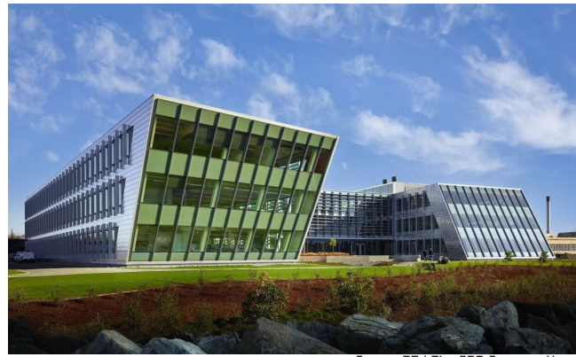
Figure 07 | The FCS Exterior View
