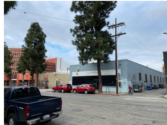
F82 | Front of small existing building
