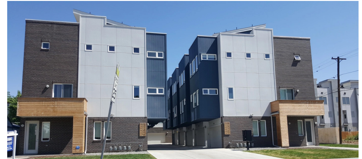
F02 | An example of an unaware building design | Denver, CO
