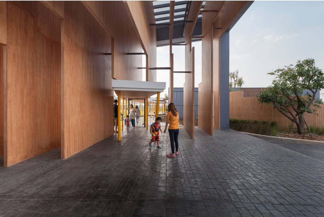
Figure 16- Rutchut School Front Facade
