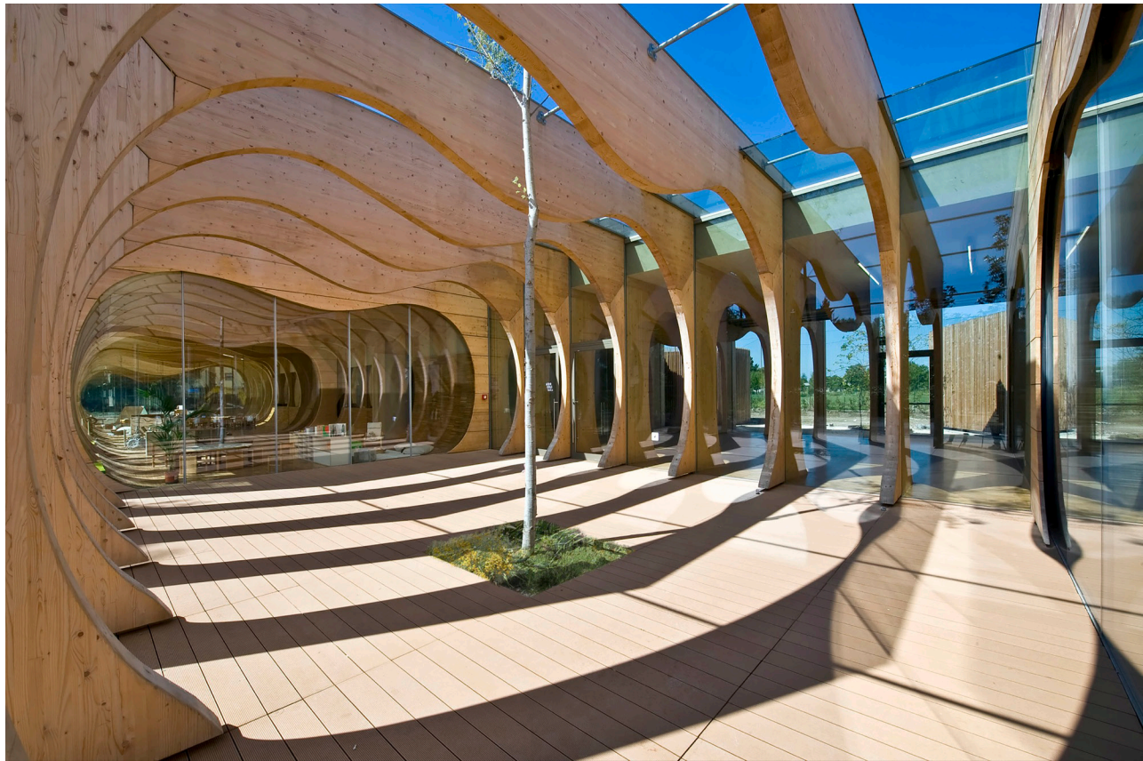
Figure 41- Kindergarten in Guastalla Material
