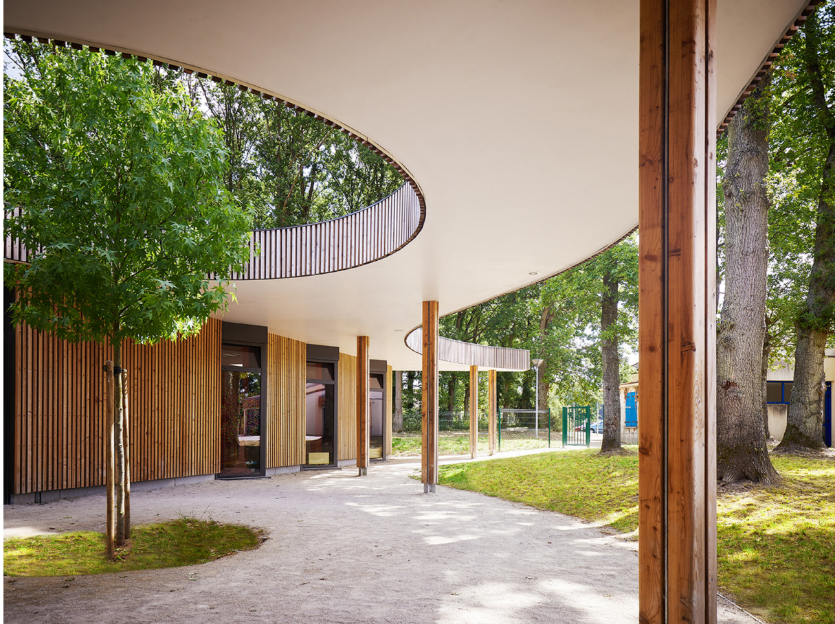
Figure 50- Children's House Roof
