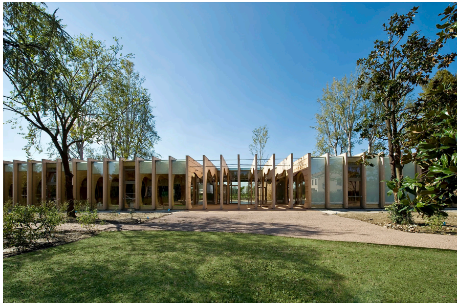
Figure 38- Kindergarten in Guastalla Exterior
