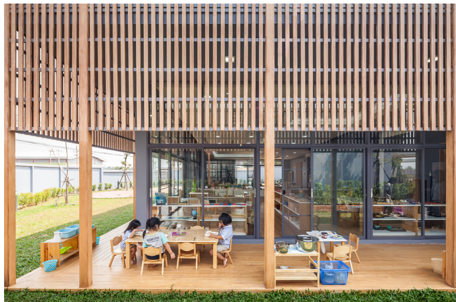
Figure 9- Rutchut School Outdoor Work Area
