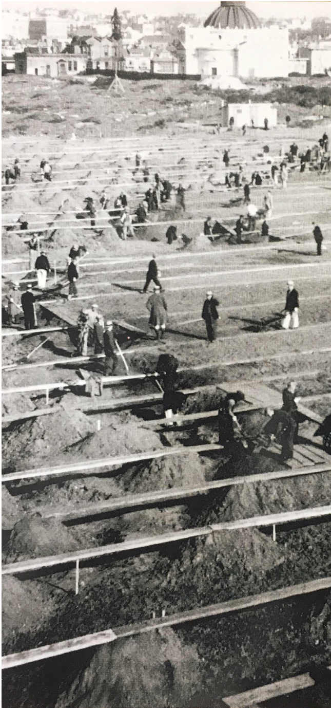
FIGURE 32 | REMOVAL OF OLD FELLOWS | SF PUBLIC LIBRARY
