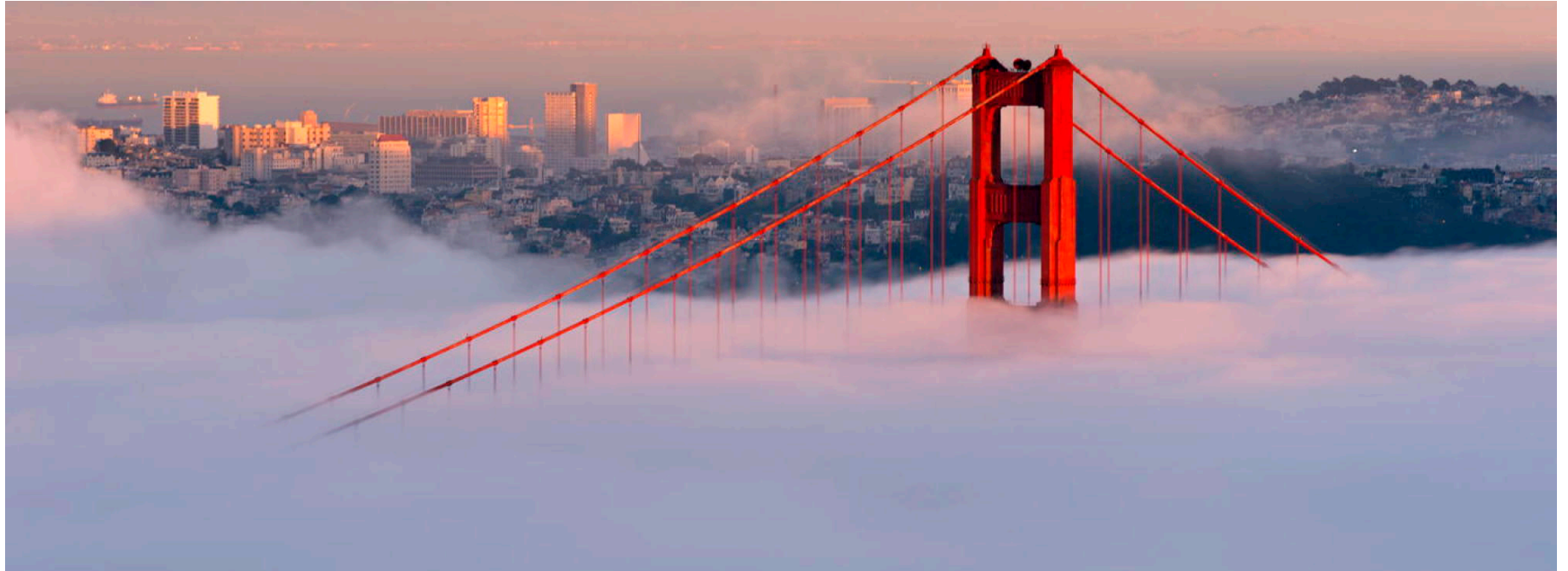
FIGURE 44 | GOLDEN GATE BRIDGE | THE PARNASSUS GROUP
