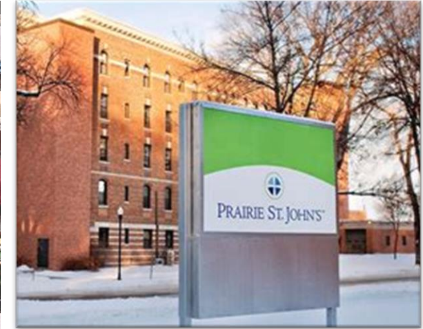
Psychiatric Hospital Facilities
