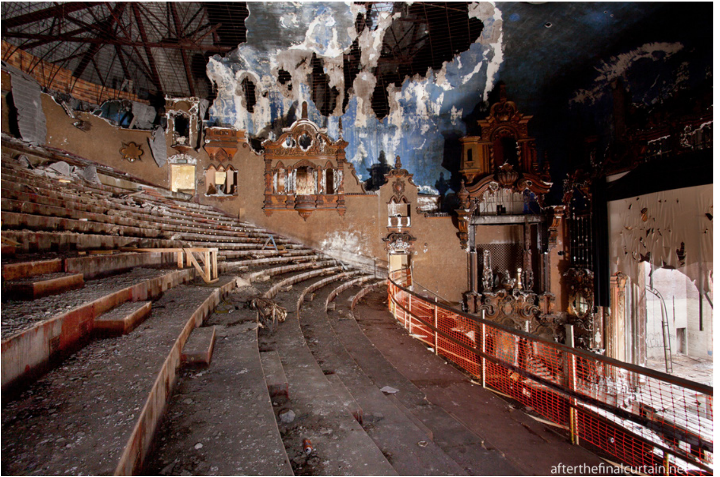
Figure 50 | Old Auditorium Space , photo credit | After The Final Curtain
