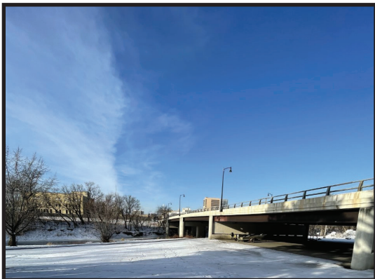
South toward NP Ave. bridge Figure 47
