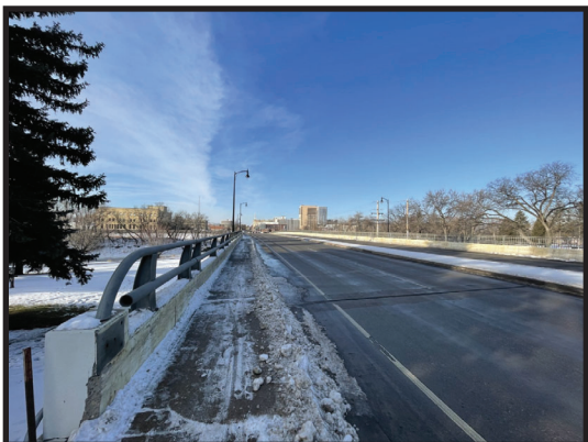
1st Ave. bridge looking west Figure 49
