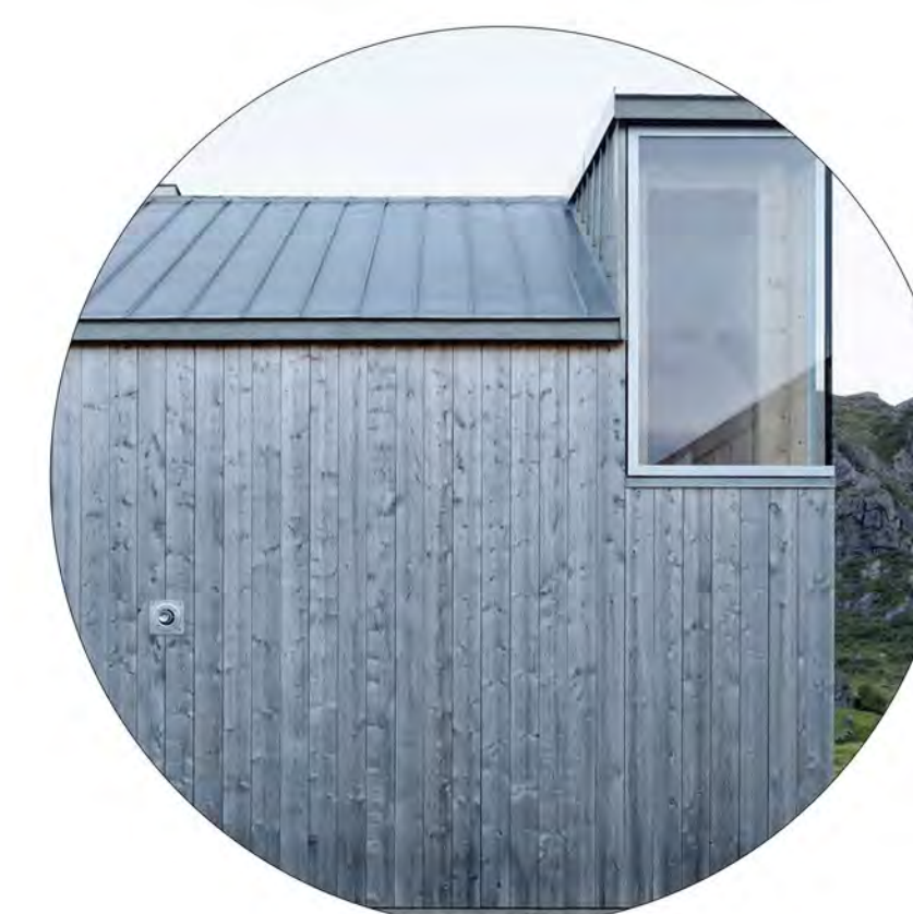
WOOD CLADDING • SOURCED FROM NEARBY SUSTAINABLE FORESTS • MINIMAL EMBEDDED ENERGY • WEATHERS NATURALLY
