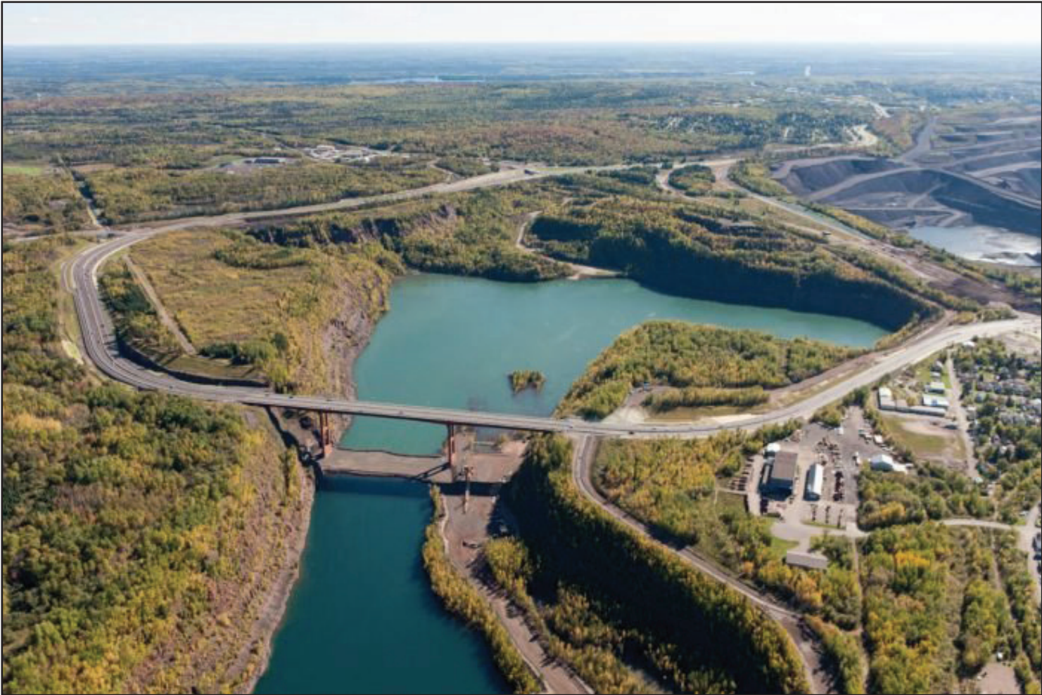
Figure 61 - Virginia High Bridge
