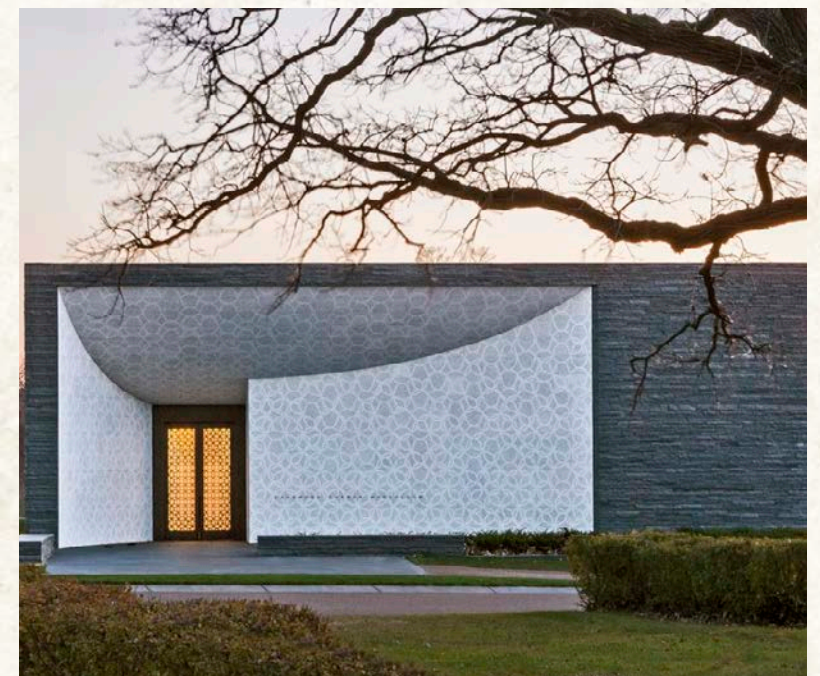
Figure 13 | Mausoleum Entrance | HGA
