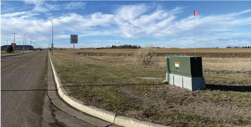
Figure 104 - SE Corner of Site 2
