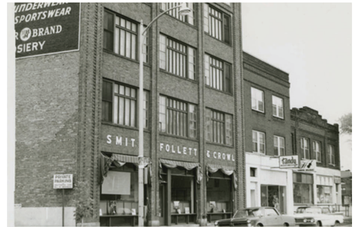
Figure 41 | Lofts on Roberts, historical front
