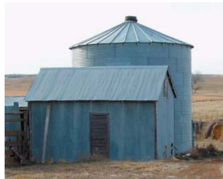
Figure 39. Existing storage buildings on site.
