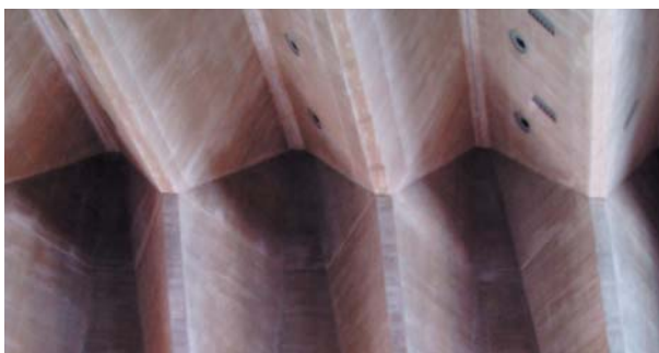
Figure 66. Interior detail of folded plates at roof/wall connection.
