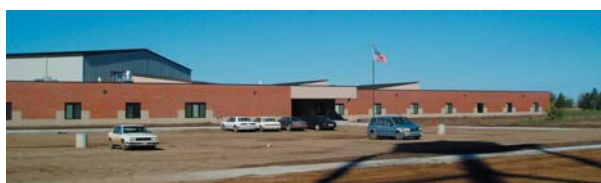
Figure 16. Bonesteel-Fairfax High school still partially under construction.
