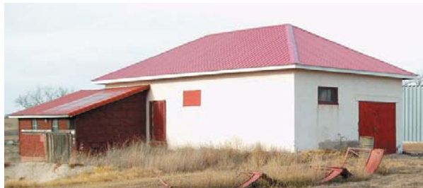
Figure 40. Existing storage buildings on site.
