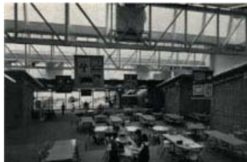
Figure 61. Light freely passes through the open members of the structure and into the spaces.
