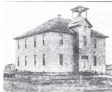
Figure 6. First public school building in Gregory.
