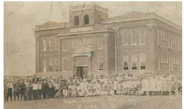
Figure 10. New brick school building.
