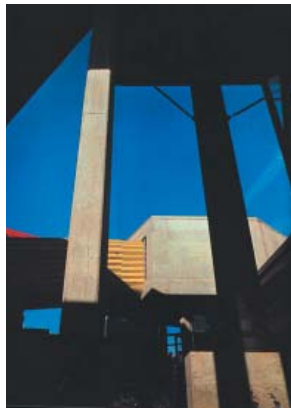
Figure 54. The bright colors of the steel corridors are accentuated further in contrast to the natural color of the concrete.
