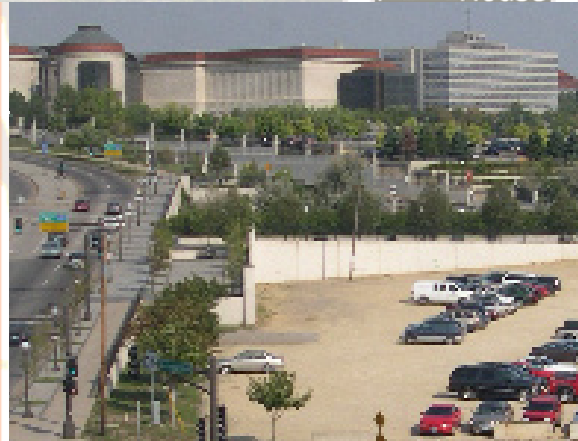
Figure: E-30 Retaining Wall
