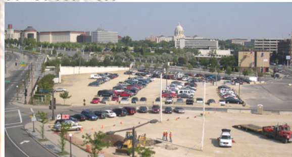
Figure: E-6 Northern Site Overview
