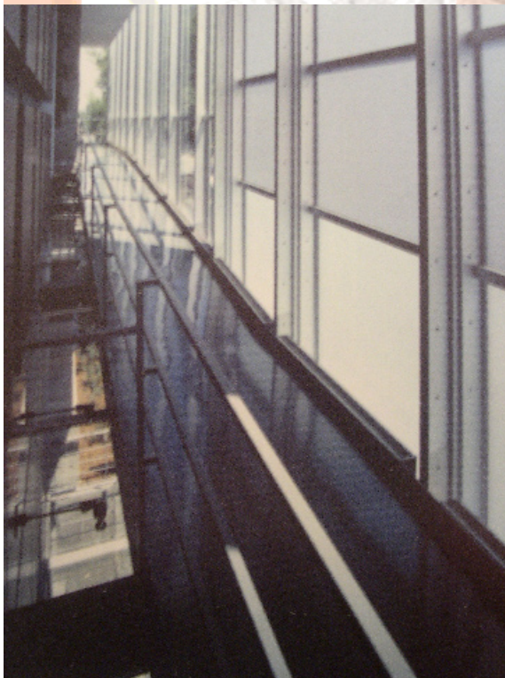
Figure: B-42 Cinematheque Quebecoise Circulation Space
