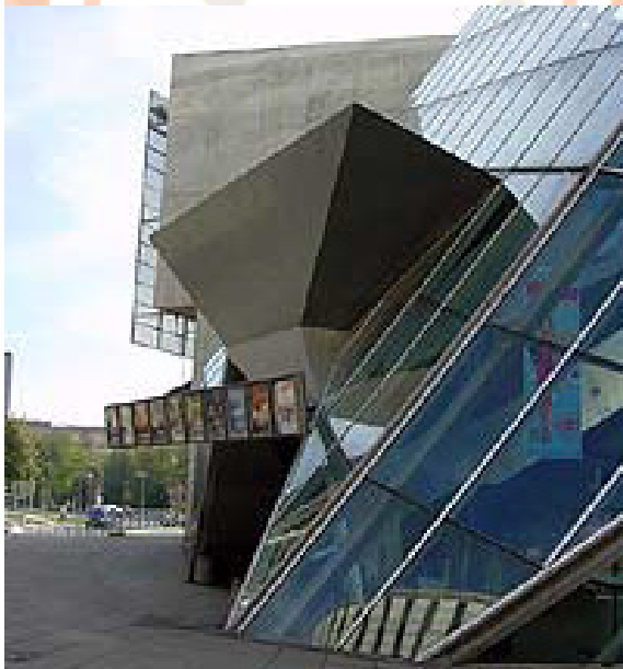
Figure: B-2 UFA Cinema Center Facade Structure
