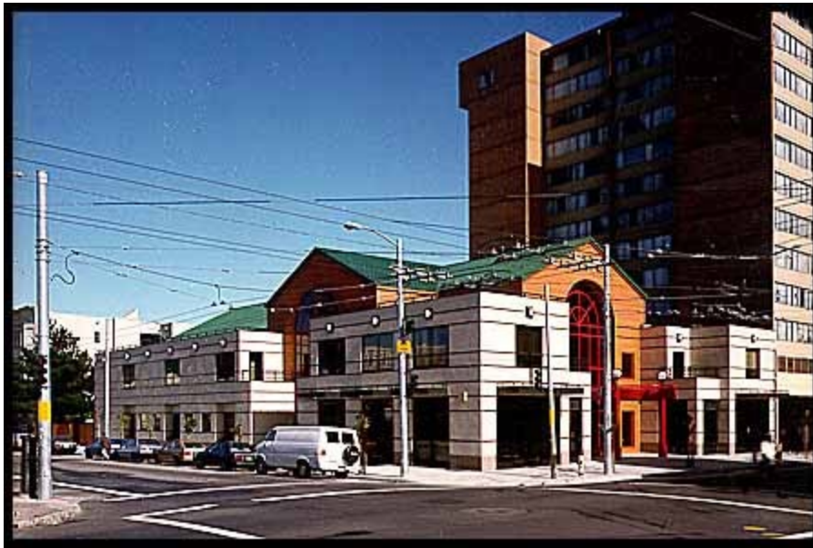
Figure 5.16 West Bay Community Center
