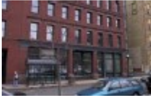
Figure 4.4 Typical Building Façade in Lowertown Neighborhood
