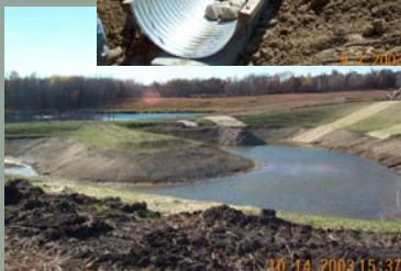
Figure 7.9 Water Aerator & Filtration Pond
