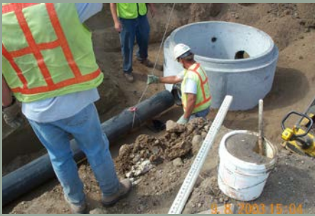
Figure 7.8 Ground Water Extraction Pump
