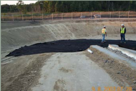
Figure 7.10 Filtration Pond Construction
