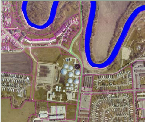
Figure 7.23 Fargo Waste Water Treatment Center ( www.cityoffargo.com )
