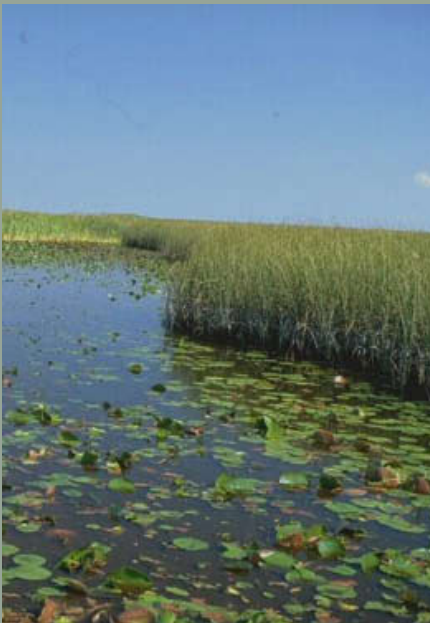
Figure 3.5 Constructed Wetland ( http://sofia.usgs.gov )
