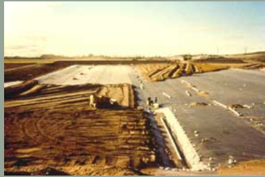
Figure 2.4 Landfill Liner (www.cityoffargo.com)
