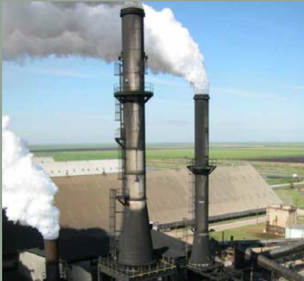
Figure 7.20 Incinerator Smoke Stack
