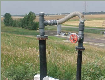
Figure 5.2 Methane Collection Pipe (www.cityoffargo.com)
