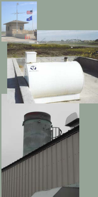
Figure 6.32 Built Structure at Fargo Landfill
