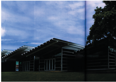
Front view of the Library. The exterior is divided into sections that have angled roofs to allow for natural daylighting and ventilation.
