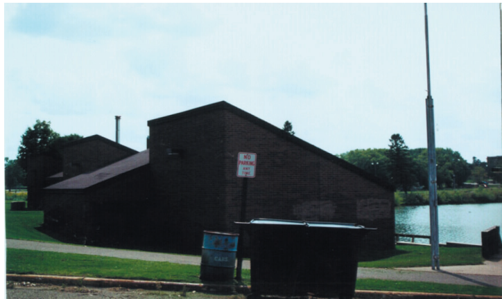
This building serves as the park shelter. It was once used as a warming house, concession stand, and rental office. It sits empty and un-used today. It is located on the East side of the lake.
