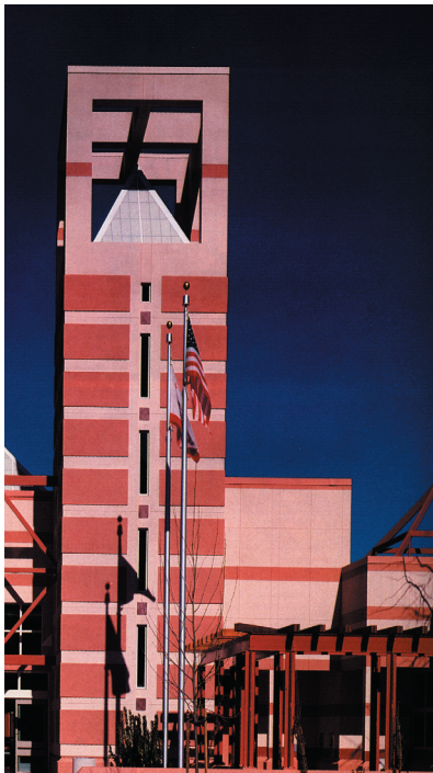
The entrance for the Albany Library and Community Center is very iconic. It visually divides the two functions.
