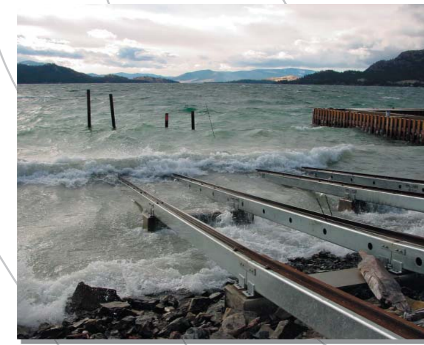
Tracks for parking the boats in the garage.
