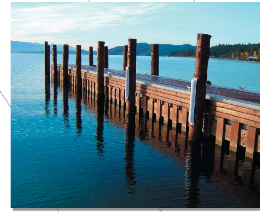
Current docking foundation on concrete pylons.
