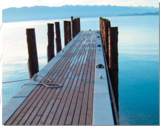
Completed Docking Facilities
