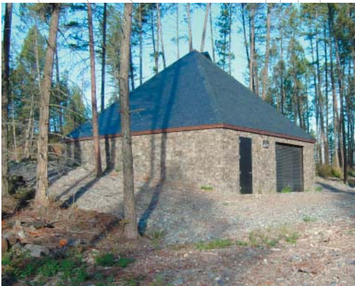
Power Station and control for the Island
