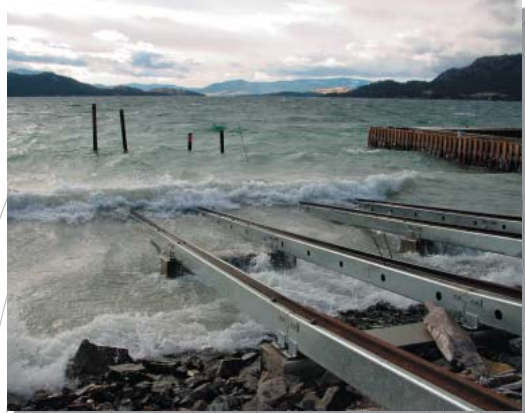
Tracks for parking the boats in the garage.
