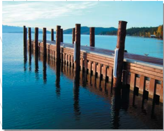
Current docking foundation on concrete pylons.
