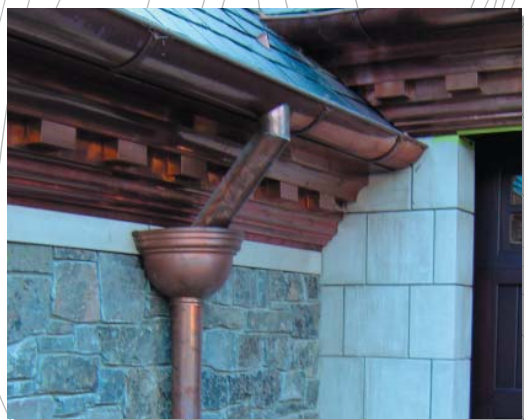
Copper accents of Gutters and Flashing
