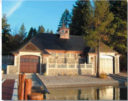
Completed Main Land Boat House
