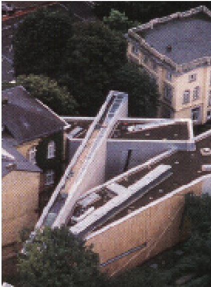
Figure O.22 FNM Aerial Site View
