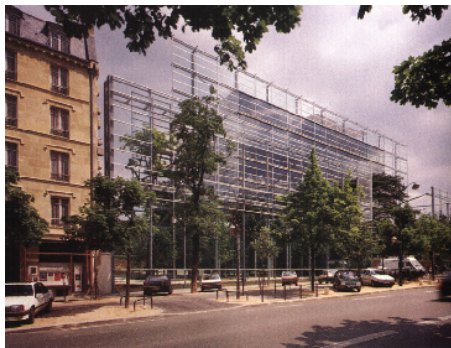
Figure O.59 CFCA Exterior
