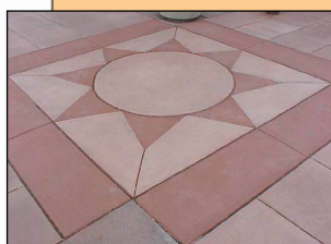
Above: Detail of sunburst pattern at intersection of walkways. Concrete colors were selected to blend with existing walls and surrounding building color schemes. ▲
