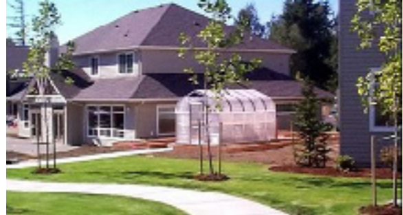
Figure 23: El Dorado Building
