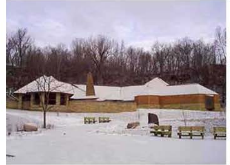
Figure 5.8. The architects for Fort Snelling State Park Visitor Center drew inspiration from Minnesota’s historic rustic park architecture
