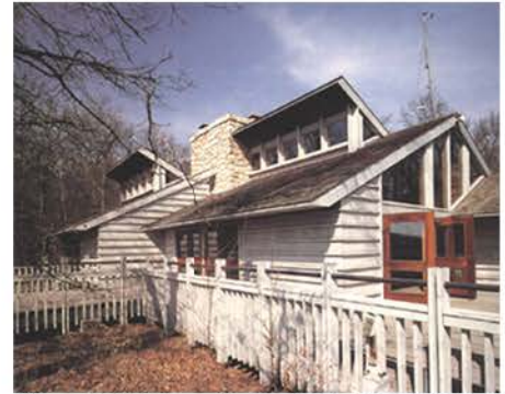
Figure 5.11. The center is oriented toward the sun with a three sided deck and clerestory windows open to the outdoors
