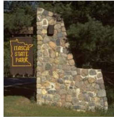
Figure 1.1. Entrance to Itasca State Park
