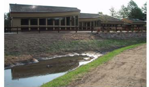
Figure 5.3. The building appears as many smaller masses in order to make it seem less
