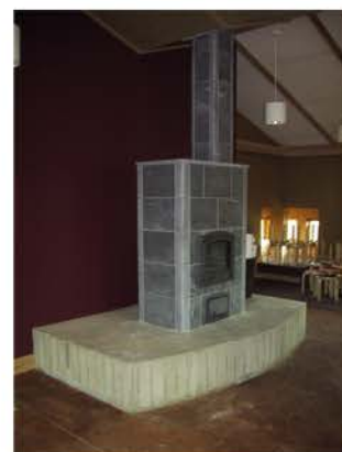
Figure 5.6. The soapstone fireplace provides heat in the building for 10 hours with just one hour worth of fire
