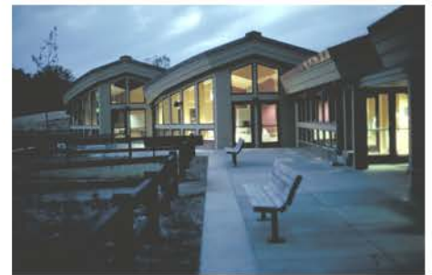
Figure 5.2. The center contains many low "E" windows which help to insulate the building
