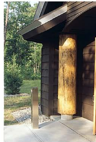
Figure 5.24. The red pine columns were fabricated from trees harvested to clear the building site
