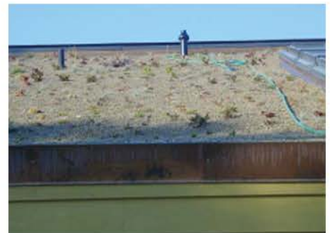
Figure 5.5. The vegetated roof increases energy savings in heating and cooling as well as helps the building blend in with the environment
