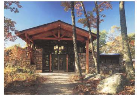
Figure 5.14. Native stone and timber are used for the entrance to reinforce the building blending in with the site
