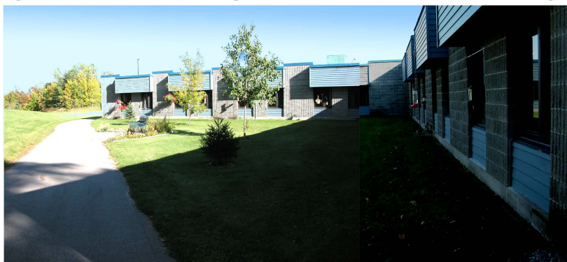
Figure 38: Walking Path Behind Resident Rooms
