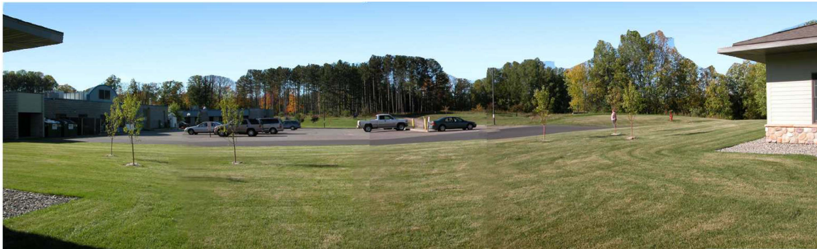
Figure 49: Lodge Back Lawn View of Parking Lot
