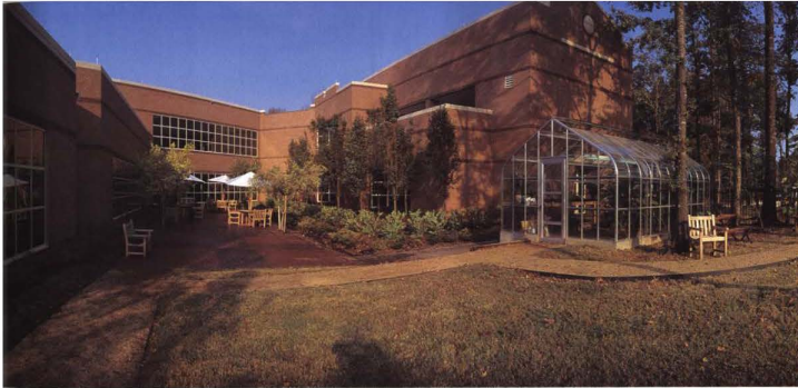
Figure 67: Courtyard at St. Michael
