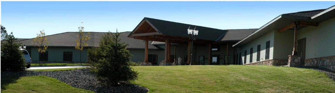
Figure 32: The Lodge Entrance from the north
