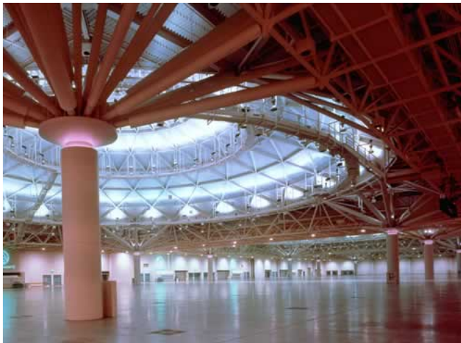
Exhibition space with iconic roof structure and other structural elements used as aesthetic qualities.
