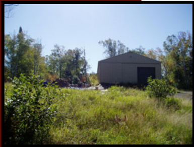
Figure 37- Maintenance Building (Schlukebier 2004)
