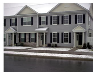
Townhouses in Chaska, Minnesota. These form a strong relationship with the street.
