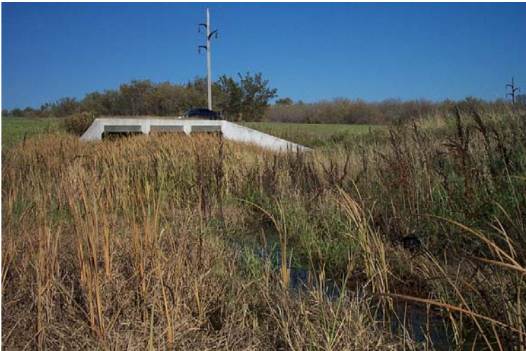
Looking north at culvert under 52 nd Av. South
