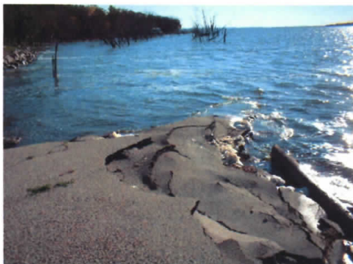
Figure 37. Old Site Road
