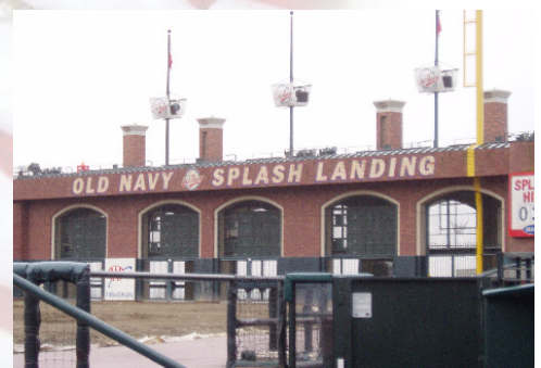
Fig. 3.16: The right field facade, with an open view for outside pedestrians.
