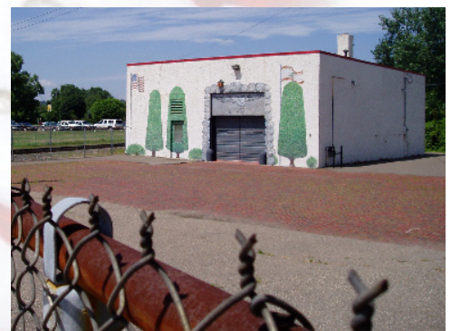
Fig. 2.30: View 3. Nasseff Plumbing & Heating Warehouse.
