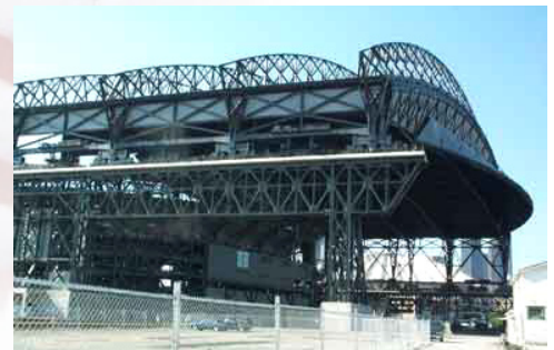
Fig. 3.11: Structure of the roof.
