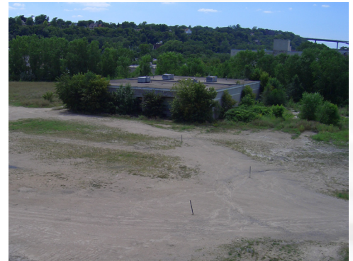
Fig. 2.34: View 1. Fillmore Ave.
