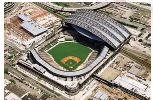
Fig. 3.9: Safeco's retractable roof.
