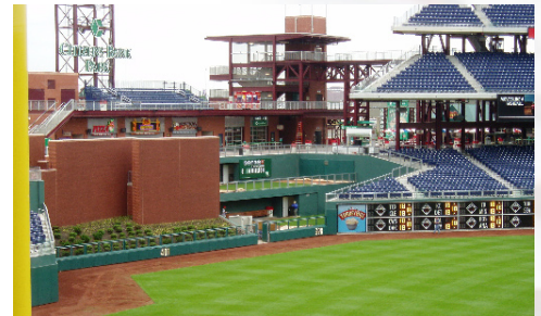
Fig. 3.3. The playing field is 23 feet below grade.
