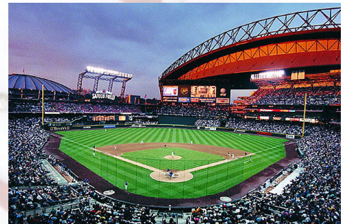
Fig. 3.10: Safeco with an open roof.
