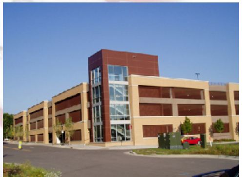
Fig. 2.33: View 3. Robert St. parking garage.
