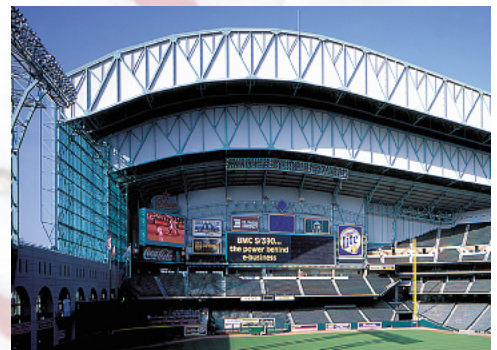
Fig. 3.13: The roof open.
