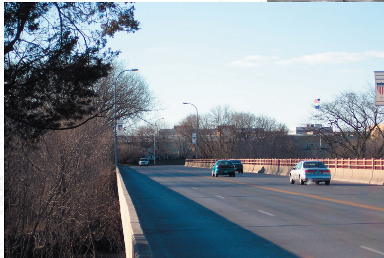
Photograph 18 Looking West Across NP Ave Bridge at Site
