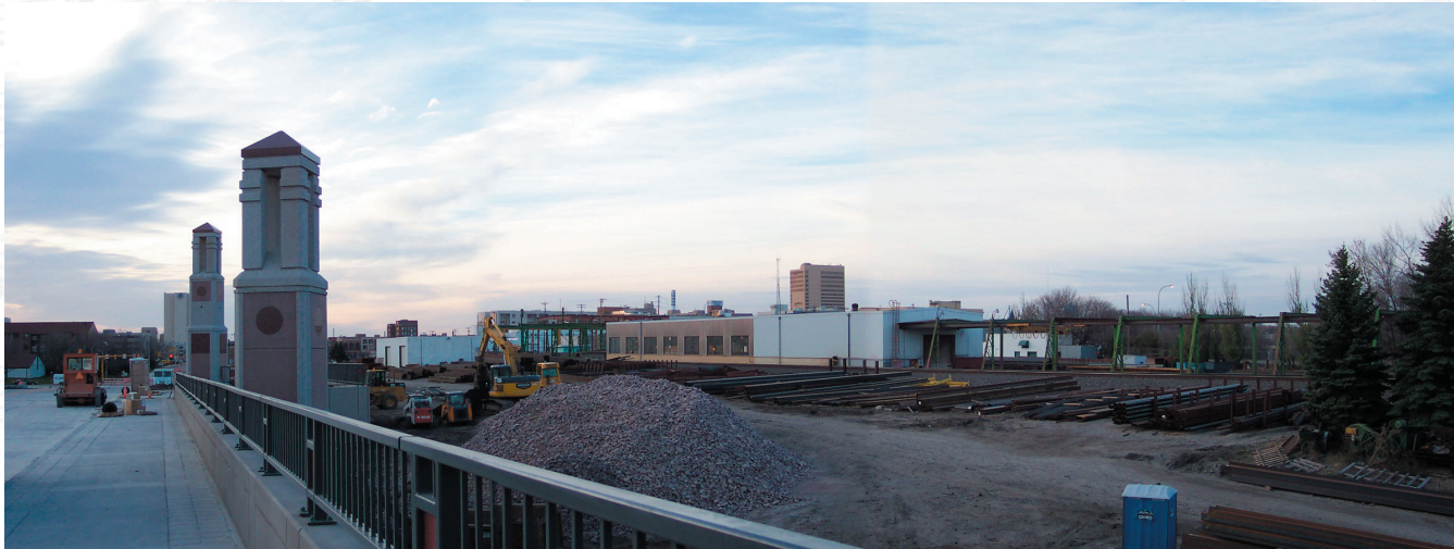
Photograph 13 Looking Down Main Ave Bridge at Site
