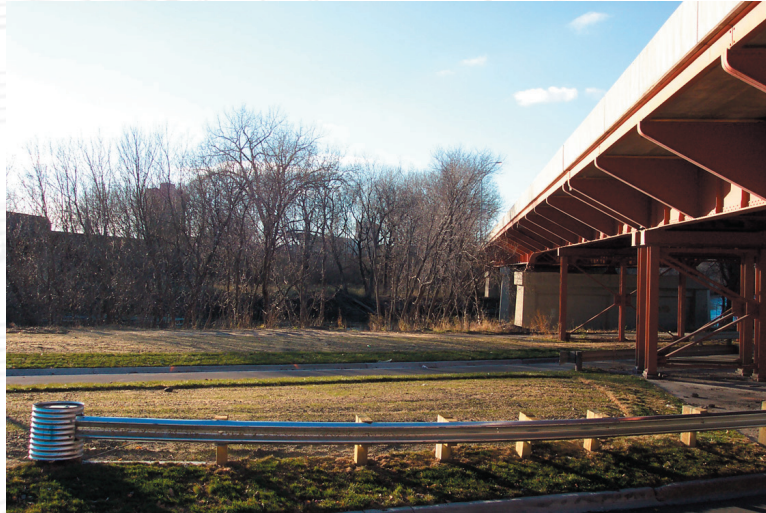
Photograph 17 Looking from Under NP Ave Bridge at Site
