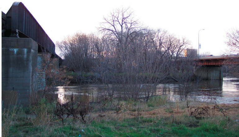
Photograph 16 Looking from the East Across the Red River at Site
