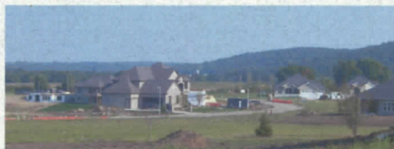
View of surrounding area to the northwest of the site
